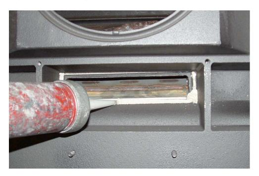
6. Starting in the bottom right-hand corner, push in the .187 gasket using a putty knife, you'll want the gasket to insert just under the fireback along the bottom edge. **Note:** You may have to use your putty knife and a hammer to gently tap the .187 gasket under the stainless steel lip of the fireback.
