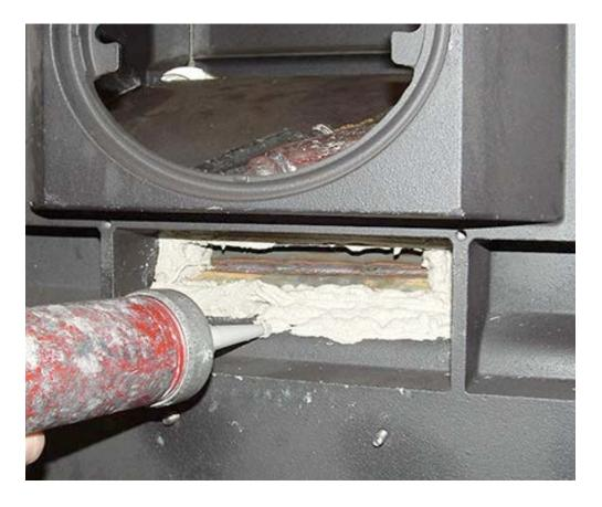
10. With wetted fingers smooth the cement, to help ensure a smooth airflow into the secondary fireback.
